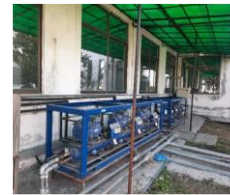
Outdoor/indoor coolers (3hp, 5hp, 7hp, 10hp)
