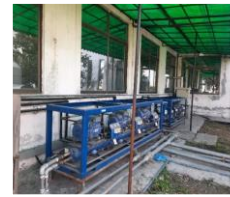
Outdoor/indoor coolers (3hp, 5hp, 7hp, 10hp)
